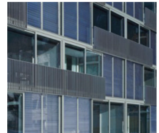
PCM-integrated facade changes translucency as the salt hydrate changes state. This phase change stores energy.
