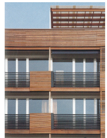
Building-Integrated evacuated tube collectors form guardrails. From Schittich 2003, 29.
