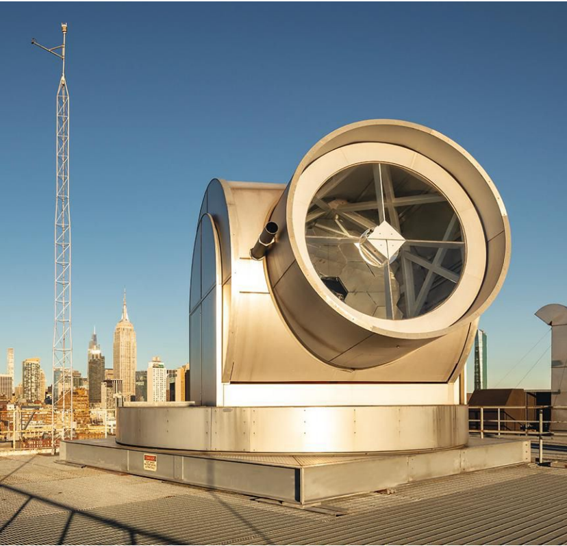
A rooftop light cannon (left) collects sunlight, directing it to a light box (above), which channels the daylight through the 208-foot-long “dagger.” Another set of optics creates a real-time image of the sun on the ceiling.
