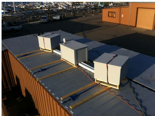
Figure 6 The test cells in place
