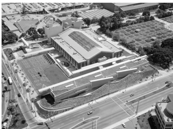
Figure 1: Aerial view of school and the open to sky courtyard in the attached armory building to the south.
