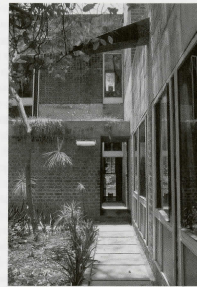
FIGURE 10. Northeast dining room and living room windows receive early morning sun in May.
