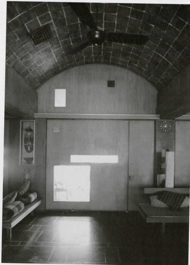
FIGURE 14. The large pivoting doors on the southwest are closed between the interior and the garden.
