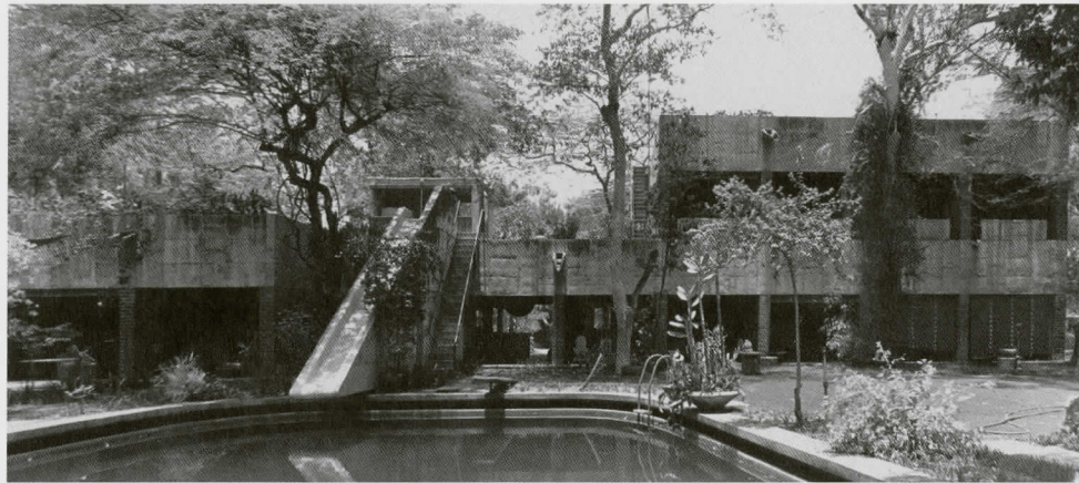
FIGURE 1. Sarabhai house, viewed from the private garden. Ahmedabad, India, 1951–54. Architect: Le Corbusier.
