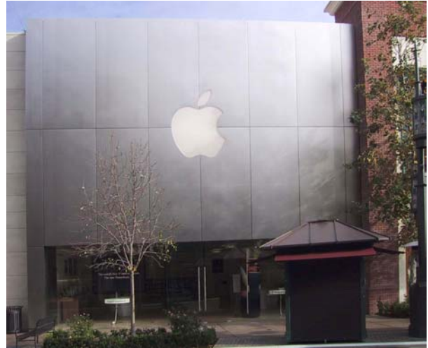
Fig. 1: Apple Store at Farmer's Grove, Los Angeles, CA. Architect: Bohlin Cywinski Jackson.
